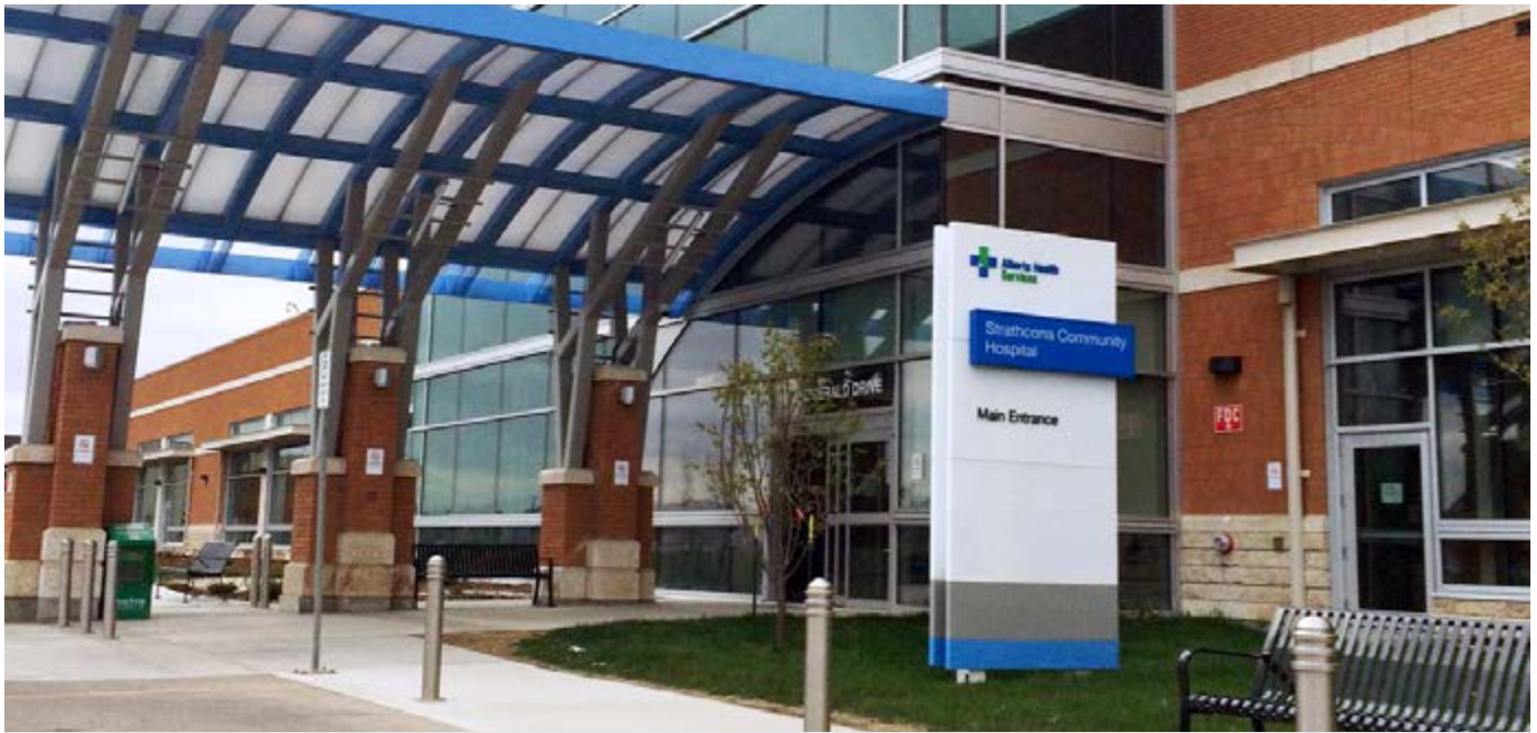
Strathcona Community Hospital is an innovative facility, delivering primary health care, combined with community-based services and a 24-hour emergency department supported by on-site diagnostic and laboratory services.
