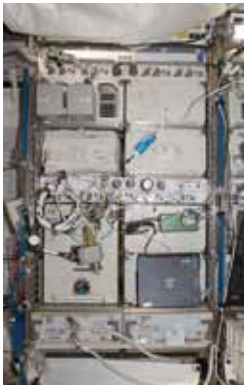
Sub-rack-sized experiments with standard utilities such as power, data, cooling, and gases.
