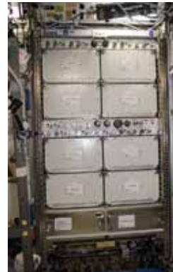
Sub-rack-sized experiments with standard utilities such as power, data, cooling, and gases.
