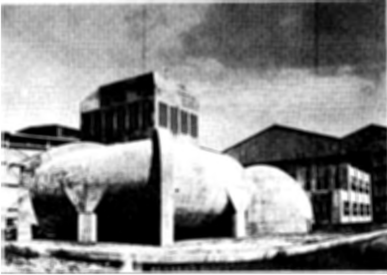
The concrete walls of the igloo-like structure around the test section of the 8-Foot High-Speed Tunnel were one foot thick.
