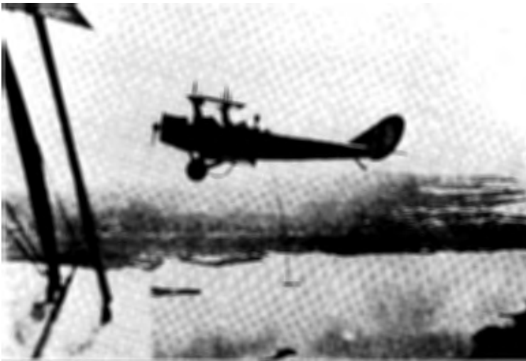
A Curtiss Jenny in flight with trailing Pitot-static tube for airspeed calibration, August 1922.
