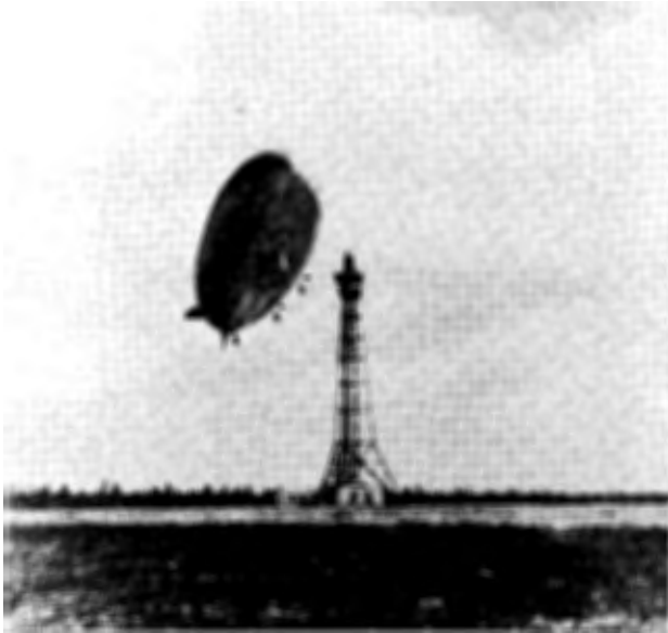
A camera obscura situated on top of a platform at the edge of the flying field measures the turning radius of the navy dirigible U.S.S. Los Angeles in 1928.
