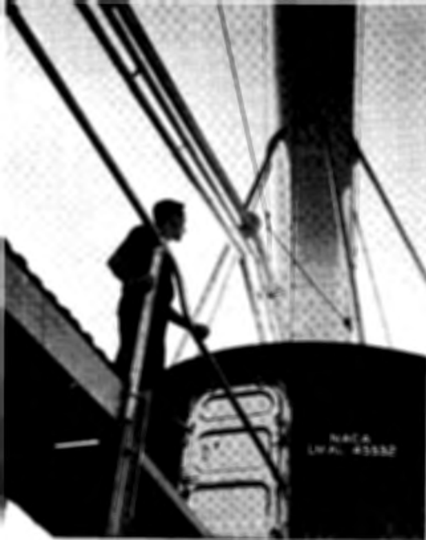
24-Inch High-Speed Tunnel.
