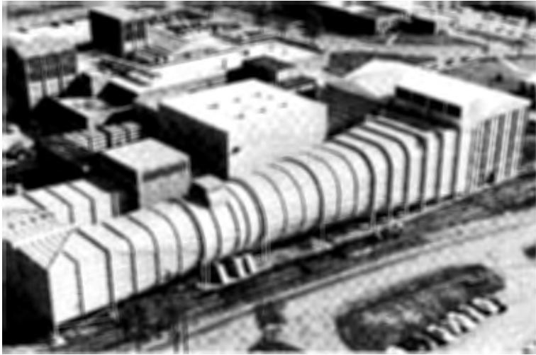
The V/STOL (Vertical/Short Take Off and Landing) Tunnel, shown here in 1949, was a modified version of the 300-MPH 7 × 10-Foot Tunnel of 1945.
