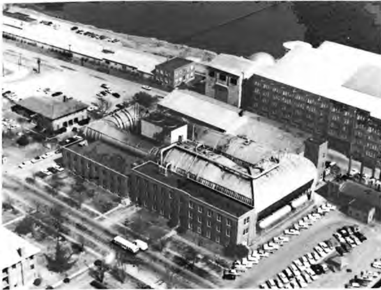
Aerial view of the Transonic Dynamics Tunnel (TDT), a greatly modified version of the original 19-Foot Pressure Tunnel. Between the TDT and the Back River stands the Full-Scale Tunnel.
