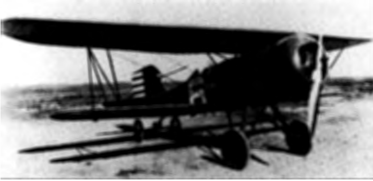
The Curtiss Hawk with NACA cowling, November 1928.
