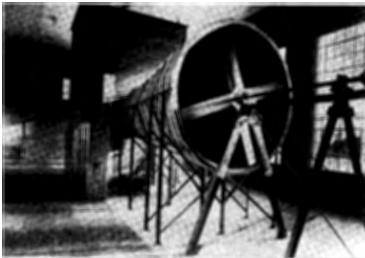
Langley's first wind tunnel, completed in 1920, was essentially a replica of a ten-year-old tunnel at the British National Physical Laboratory.
