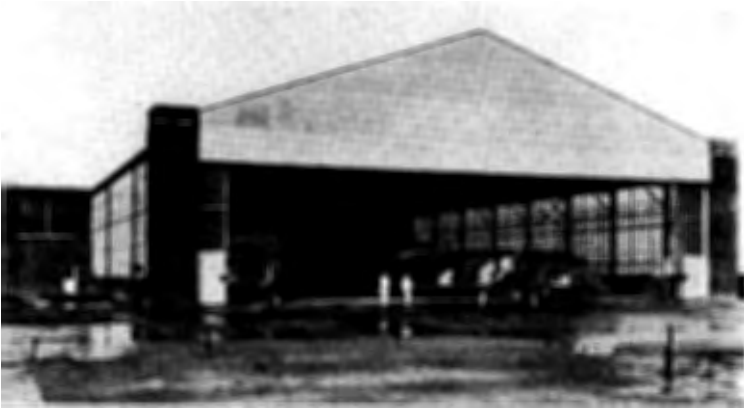
The NACA's new hangar in the east area, 1932.
