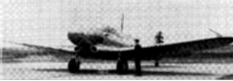
In the summer of 1939 the NACA tested an experimental cowling and cooling system on Northrop's A-17A attack plane.
